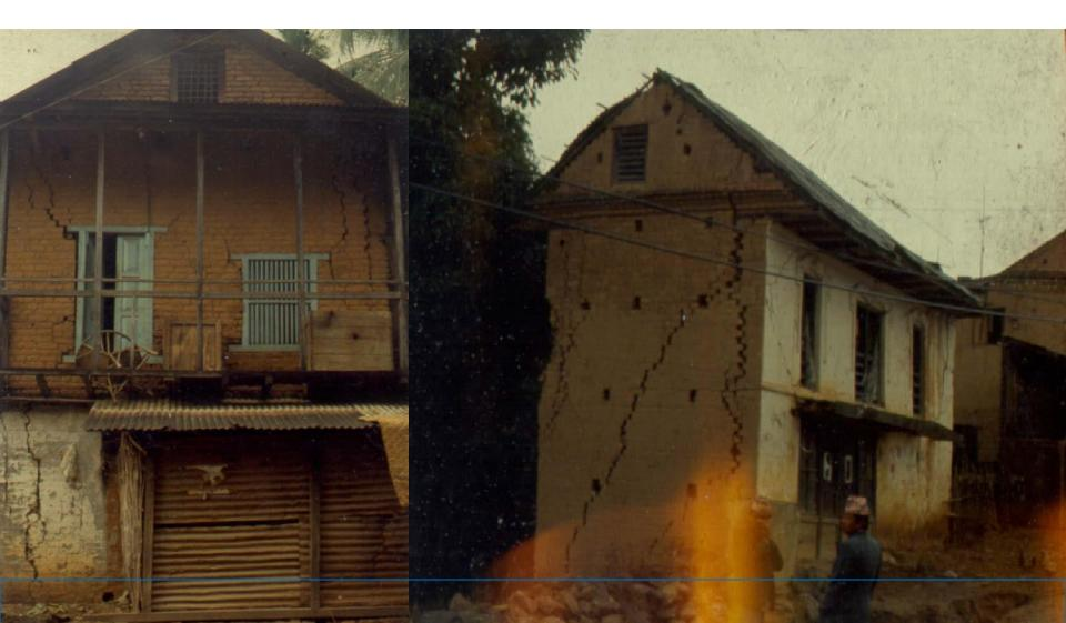
**Damage on masonry buildings start from corner separation**
