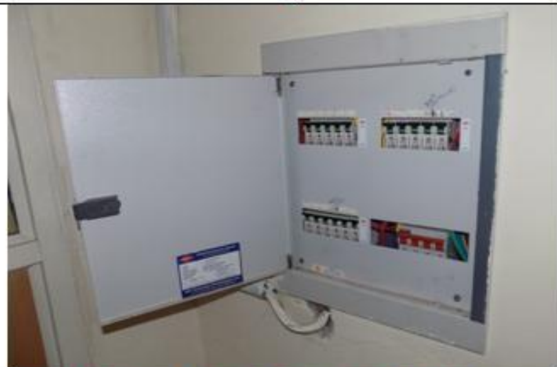
Miniature Circuit Breaker's (MCB's).
